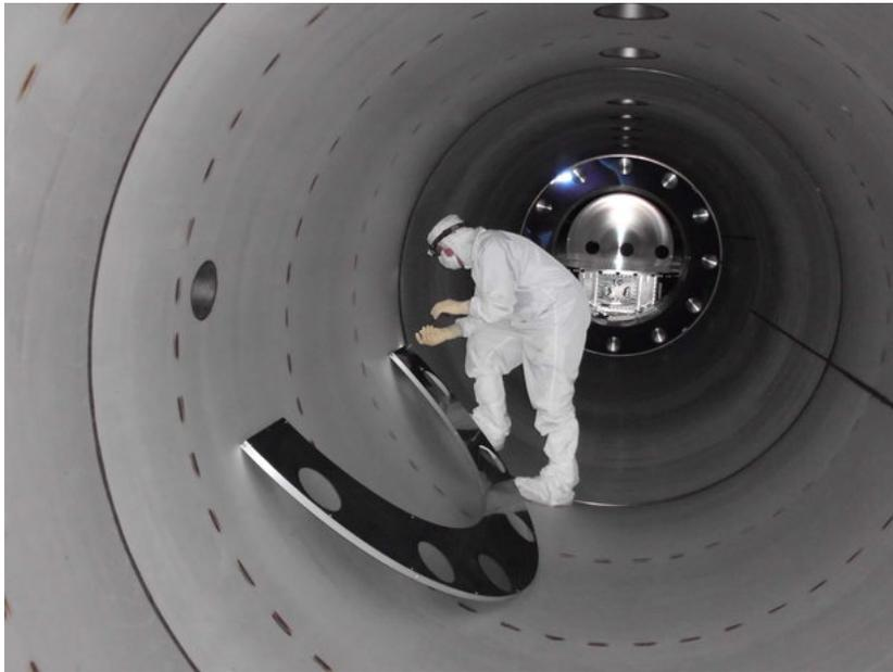
Figure 4.3: Looking down one of the long vacuum tubes that house the optical elements of LIGO during installation of the light baffles. Credit: Caltech/MIT/LIGO Lab
